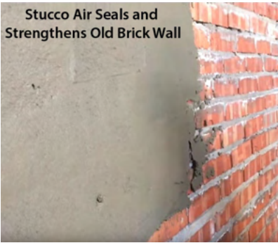
Stucco over brick: This retrofit serves two purposes: air sealing and structural reinforcement.
